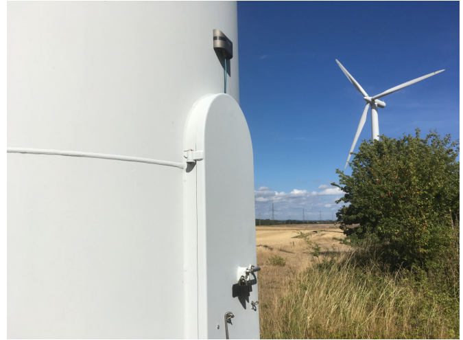
Sensor mounted above wind turbine door
