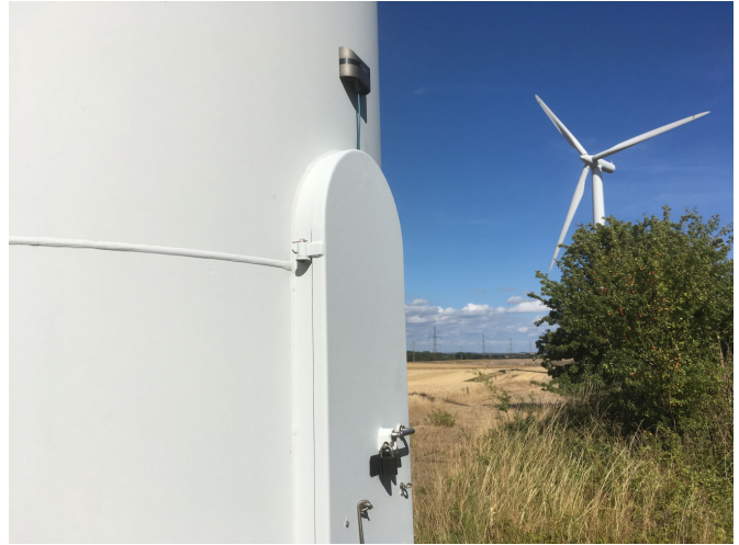
Sensor mounted above wind turbine door
