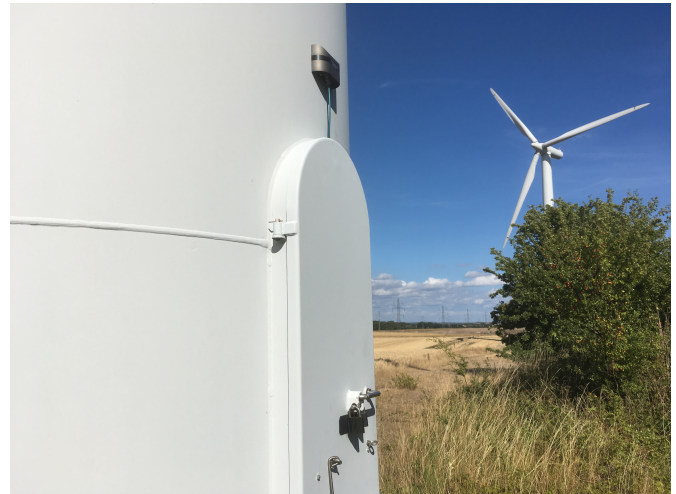
Simple mounting of sensor above wind turbine door
