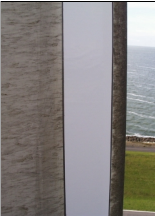
The lightning protection tape mounted on a Dutch turbine.
