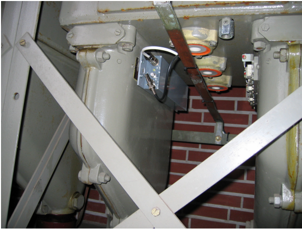
Figure 15, Re-roll having a current sensor
