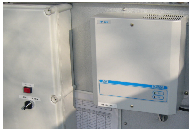
Figur 1, 24V forsyning i station (HEF)
