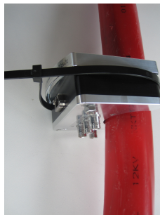
Figure 10: Complete the cable tie connection.
