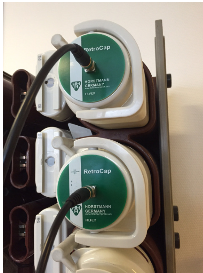
Figure 14: Horstmann RetroCaps mounted on Magnefix switchgear.
