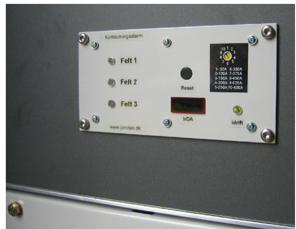
Figure 9, Short Circuit Indicator for ABB Combisensor
